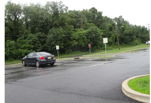
To manage parking lot runoff, parking spaces in the northeastern corner of the parking lot can be converted to pervious pavement. A preliminary soil assessment suggests that the soils have suitable drainage characteristics for green infrastructure.
