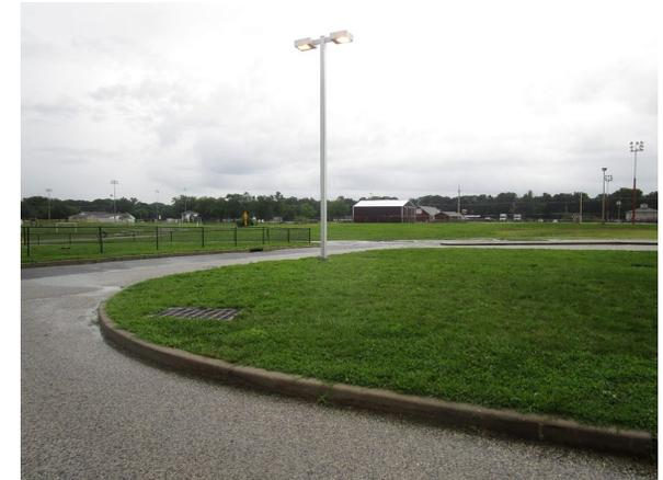
Three downspouts at the southwest corner of the building can be disconnected to a section of pervious pavement parking spots to treat and infiltrate the stormwater runoff from both the building and parking lot. A rain garden can be installed in the eastern island to capture, treat, and infiltrate parking lot runoff. A preliminary soil assessment suggests that the soils have suitable drainage characteristics for green infrastructure.
