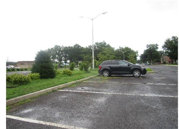
A section of parking spaces on the north side of the parking lot can be replaced with pervious pavement to capture parking lot runoff. A rain garden can be placed in the western section of the island to capture, treat, and infiltrate the parking lot runoff. A preliminary soil assessment suggests that more soil testing would be required before determining the soil's suitability for green infrastructure.
